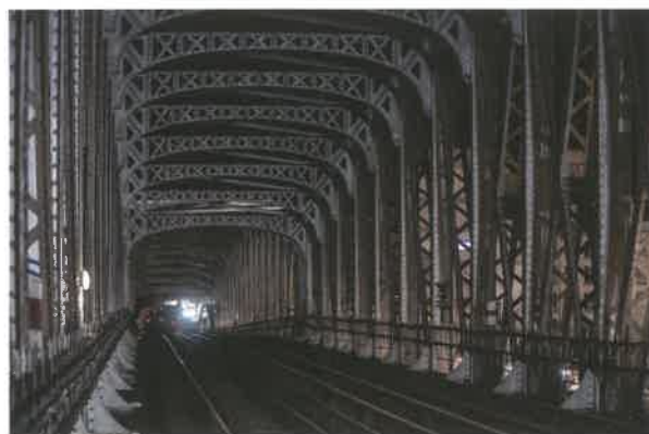
Track-related asset management
