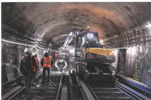
Planning and realising metro work sites
